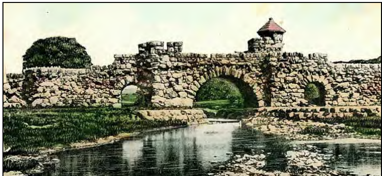
Bridge immediately behind Gate House.
